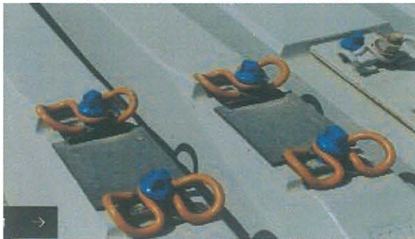
Illustration 3. Vossloh Tension clamp
