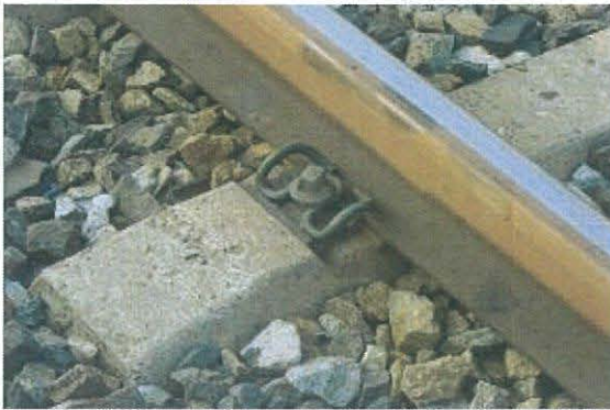
Illustration 3. Vossloh Tension clamp
