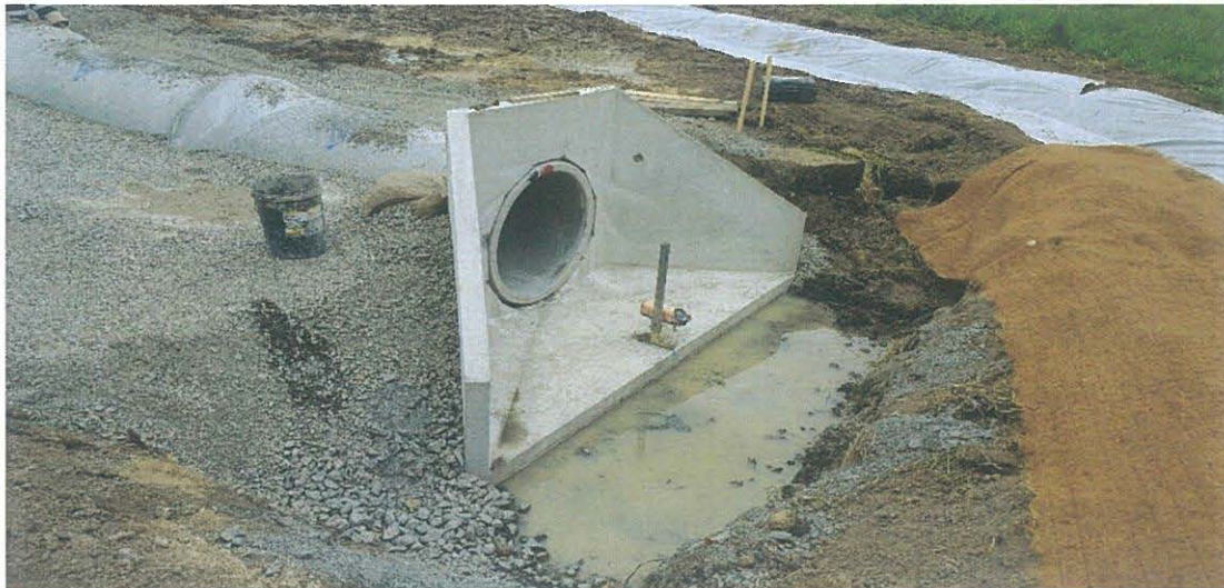
Figure 20.2 Typical Culvert End Arrangements – Pipe Culverts
